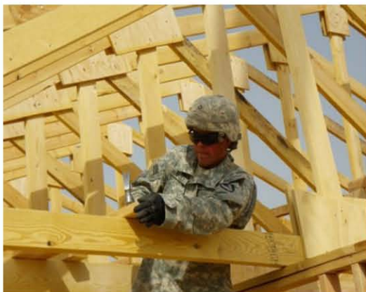
Left: SPC Amirault (2nd PLT) nails in a brace for the trusses Center: SPC Vculek (Maintenance) receives a handshake from the commander congratulating him on his promotion to SPC Right: SPC Sarlitto (2/15) operates the grader with great skill and attention to detail as he prepares the ground in preparation for the motorpool pads.
