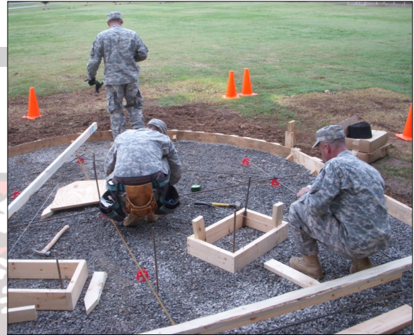
Soldiers from the 538th Concrete Detachment prepare formwork for the 5th Special Forces Group 9-11 Memorial Pad.
