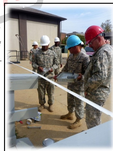
Below: Soldiers complete work on handicap ramp project
