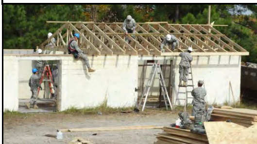
Above: 2nd Platoon renovated a storage building at Ames Range. The renovation included a new roof, electrical work, and minor masonry upgrades
