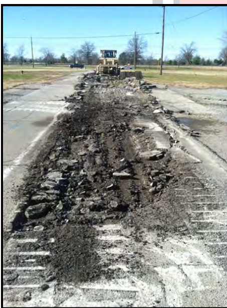
Above: A dozer breaks ground at the 2nd PLT Warehouse District Project.
