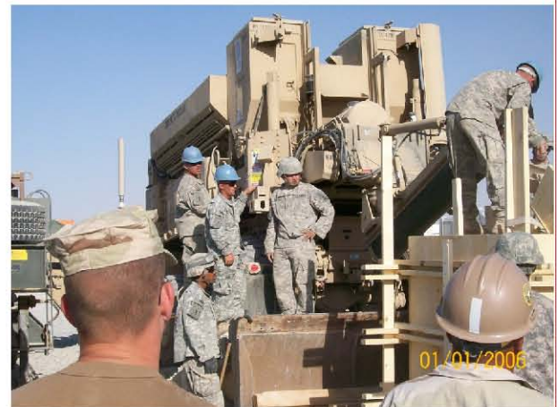
Below: Soldiers working together with the concrete modules
