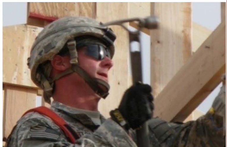
Above: SGT Norton working on installing trusses
