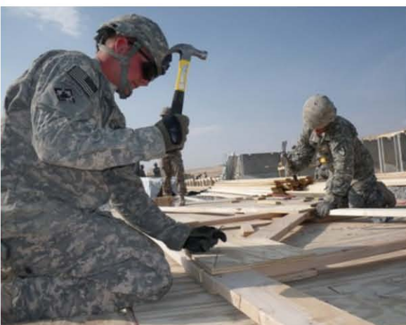
Above: 1/60EN works on building trusses
