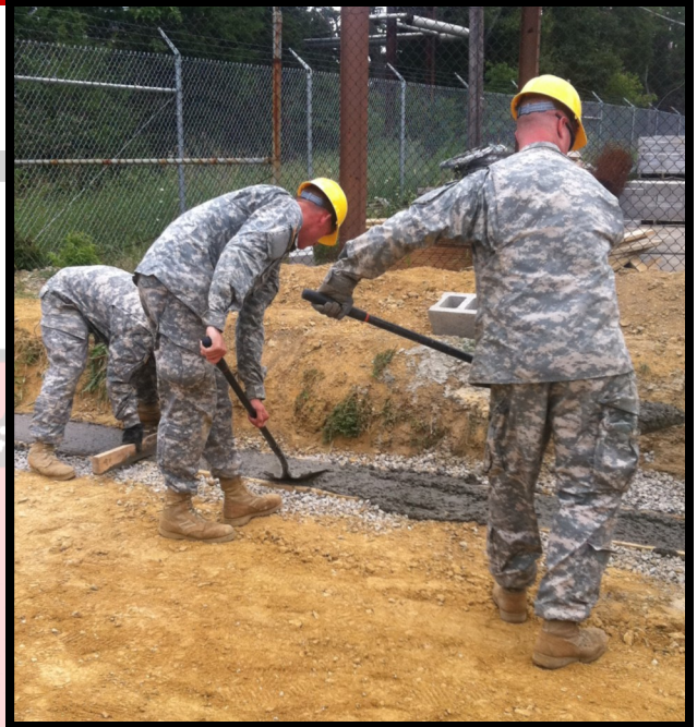
Soldiers from the 538th Concrete Detachment place concrete for a pad in the motor pool.
