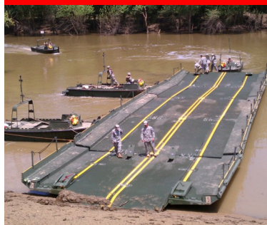
Above: The 502 assemble a float bridge on the Salt River.
