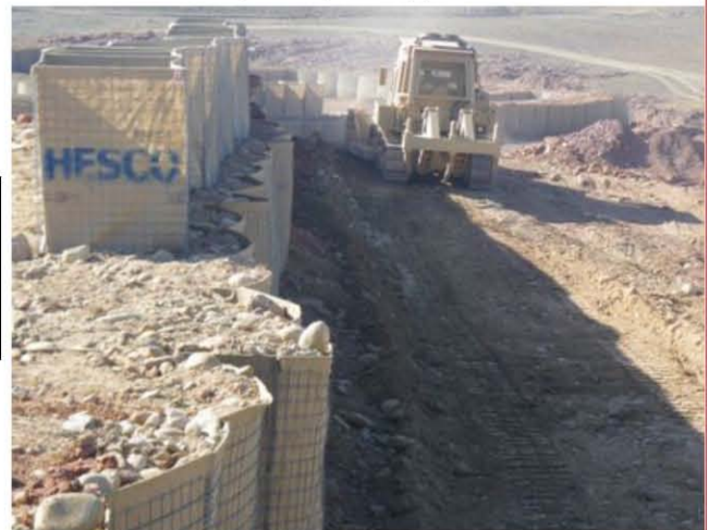
Right: 2/15 continued construction on the AHA/ Landing Zone at FOB Frontenac.
