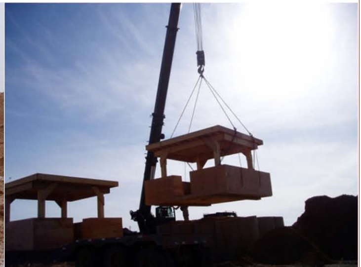
Right: 15th EN CO emplacing guard towers at FOB Delaram II.
