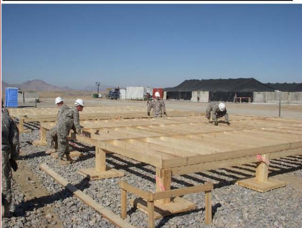
Left: 2nd PLT putting together a floor system for a future Counter IED building.
