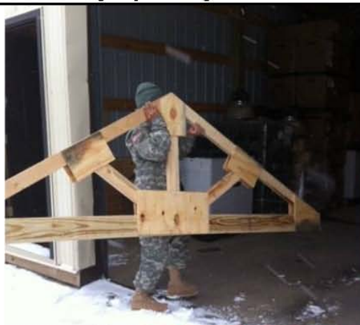
2nd PLT did a great job building some trusses in JAN
