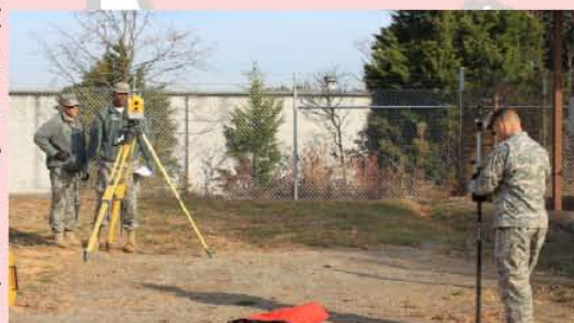
SPC Collins holds the range pole for a survey.
