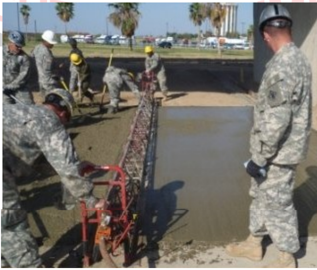
Soldiers from 1/76E pour concrete in Laredo, Texas. The Soldiers built the Border Patrol-Laredo Sector a parking lot and boat ramp
