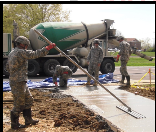
538th Soldiers put finishing touches on the sidewalk at Barr Library
