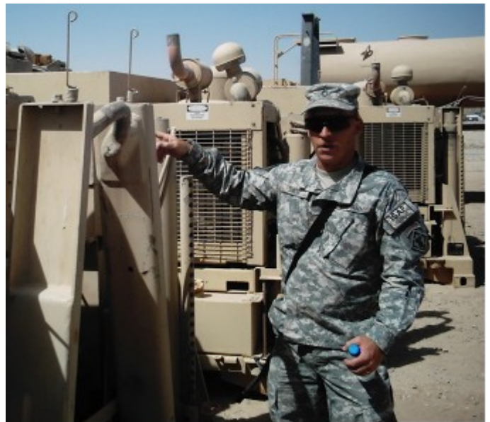
SSG Smith points to the universal rotary girder joint on a piece of equipment during a knowledge check.
