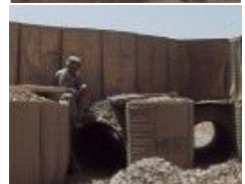
Bottom Right: SGT Poucher works to place culverts at the ECP.
