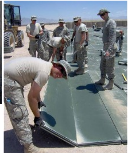
1 st PLT Soldiers working hard placing AM2 Matting at FOB TK while Chaplain McDonald provides religious support.
