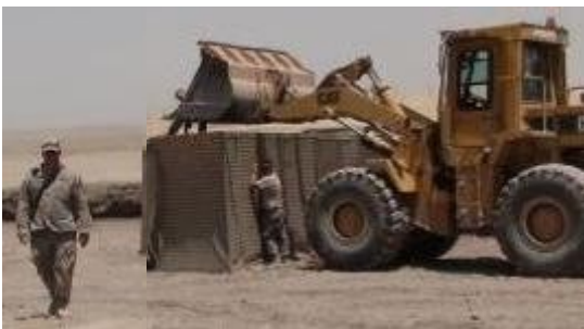
Top: SSG Allison and crew construct the vehicle loading ramp area. Right: SFC Bryant directs the crane removing a guard tower.
