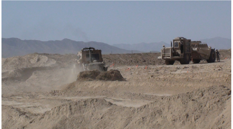
3rd Platoon's Dozers and Scrapers working hard on the ECP.
