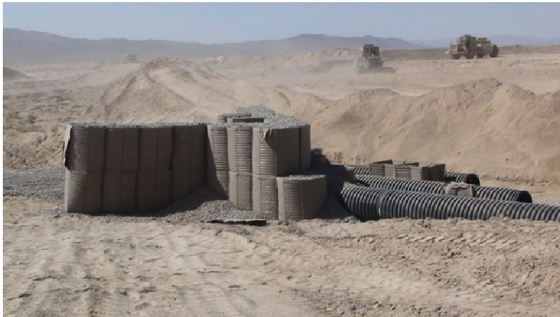
Culvert installation project to improve drainage.
