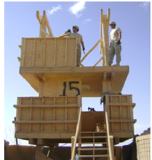
15th Soldiers use their carpentry expertise to build a guard tower.
