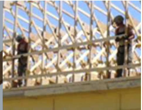
Above: Two Soldiers brace trusses on the Med Annex roof project on KAF.
