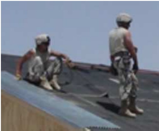
Top Left: SPC Hodgeman and SPC Kolbek work on placing tin on the roof of the SEA-hut. Top Right: PFC Mosley and PFC Johnson place footer pads on the newly compacted soil for the hut their platoon is about to build.
