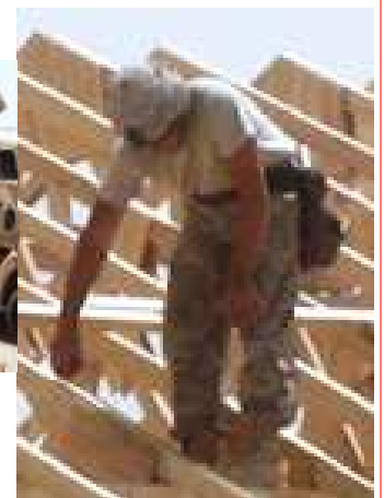
Bottom Right: SPC Leibach snaps a chalk line in preparation for nailing the plywood on the roof.
