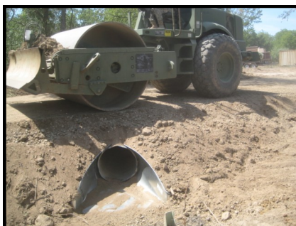
Left: SPC Prosser completing the final compaction on the road covering their newly installed culvert during the Village 62 Realism Project, Camp Atterbury.
