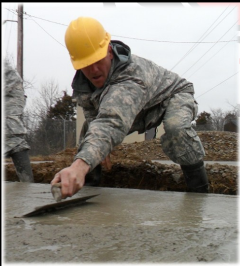
SPC Stolar trowels fresh concrete in Hurley MP.
