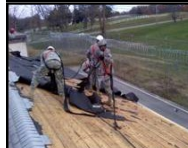
Below: Soldiers from 1st Platoon rebuilding a roof in the former post correctional facility for use by DPW.
