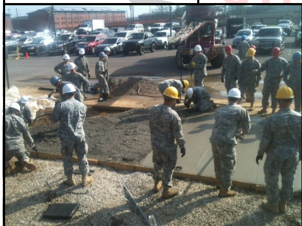
Below: Soldiers from 3rd Platoon placing concrete for the main pad of the 11th Aviation Memorial.
