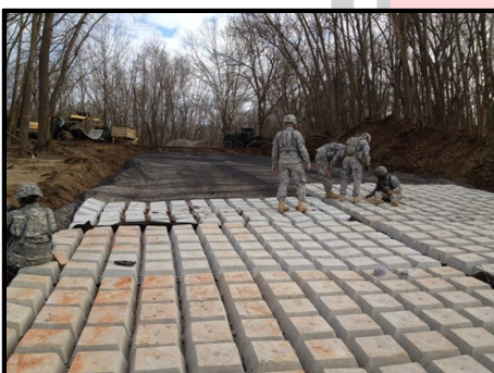
Above: 3 rd PLT Soldiers installing concrete articulated matting at the Pilcher's Landing Boat Ramp.
