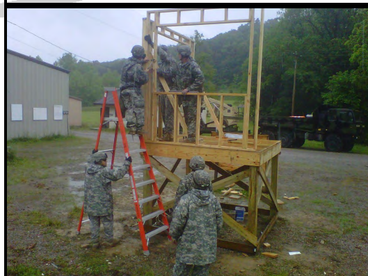
Below: 2 nd Platoon, 76 EN CO emplaces wall systems for the new tower at Choate Range..
